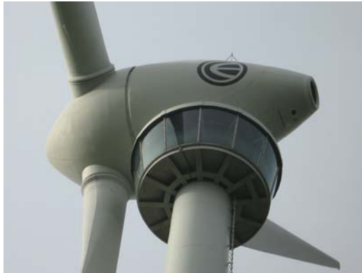
Swaffham 1.5MW turbine with viewing platform
