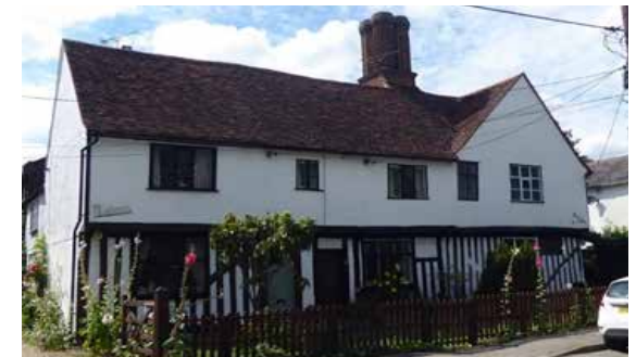
Figure 62 Exposed framing at 35 and 37 Church Lane, dating to the early sixteenth century
