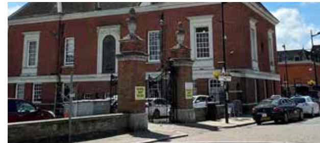
Figure 65 Walls and railings, Braintree Town Hall
