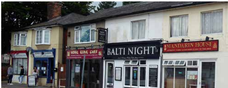
Figure 64 Shopfronts requiring improvement, Manor Street
