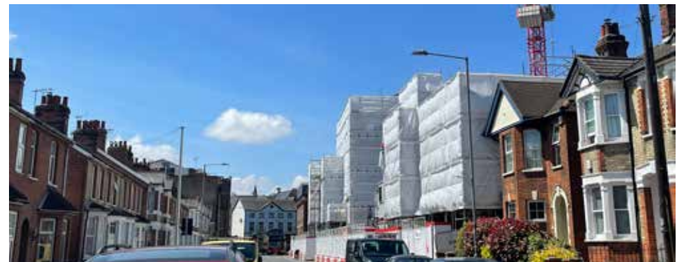
Figure 102 Manor Street development under construction, summer 2021
