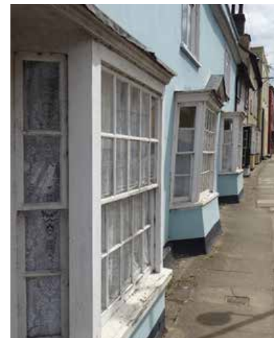
Figure 63 Bay window shopfronts added to a refaced sixteenth to seventeenth century building, 54-56 Bradford Street.
