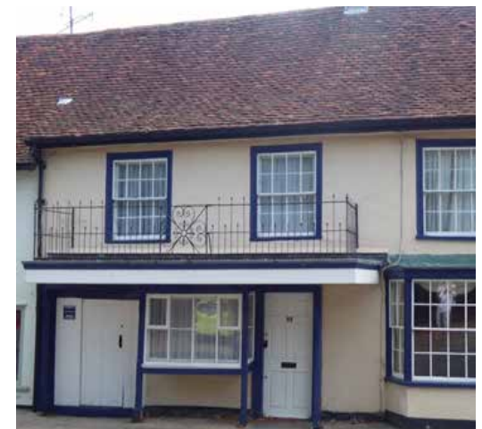
Figure 64 An eighteenth-century bay shop window on posts with a canopy in seventeenth century building at 92 Bradford Street
