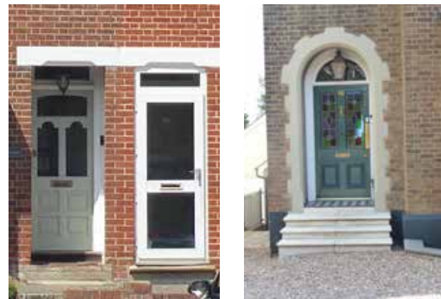
Figure 38 Examples of doors within the Character Area
