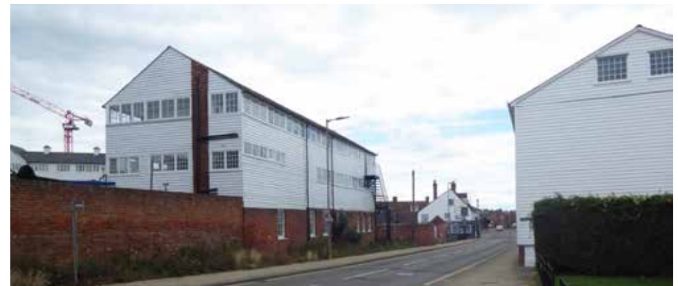
Figure 74 New Mills (left hand side) and Pund End Mill (right hand side), all Grade II listed
