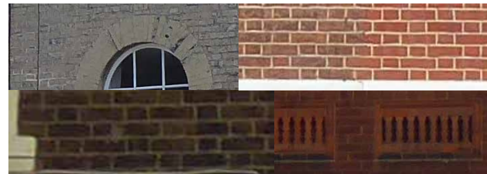
Figure 34 Examples of brickwork in the Character Area
