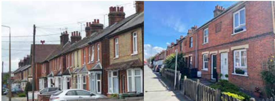
Figure 15 Terraced houses on Rayne Road, now within the Conservation Area
