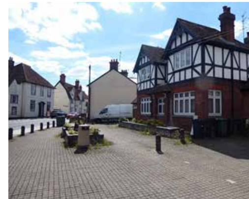
Figure 45 The small public piazza area in front of the former Six Bells at the junction of Bradford Street and Church Lane
