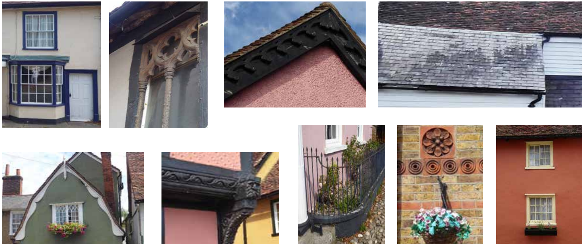
Figure 66 Top row, left to right: Nineteenth century bay window; Medieval window; Decorative bargeboards; Example of slate and clay roof tiles. Bottom row, left to right: Decorative bargeboard; Intricately carved external timber framing; Iron railings; Inset decorative clay tiles; Horizontal sliding sash windows.
