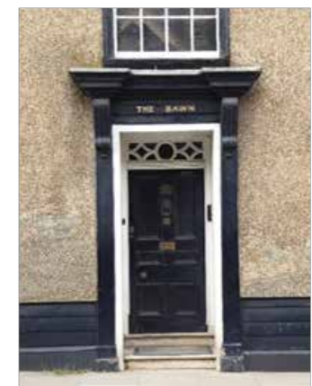
Figure 27 An eighteenth-century door, 37 Bradford Street
