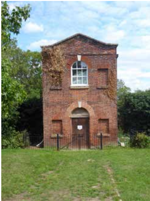
Figure 17, The Folly, St James' Road, now within the boundary.
