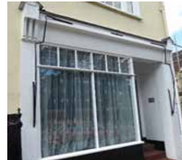
Figure 61 A nineteenth century shopfront at 15 Bradford Street
