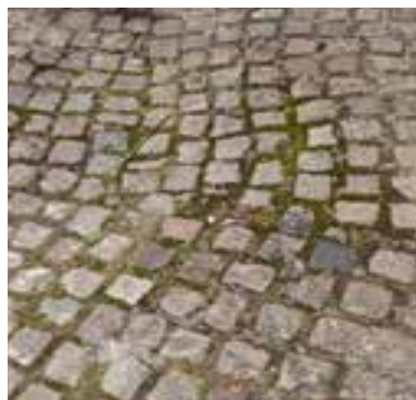
Figure 84 Example of granite setts within the pavement
