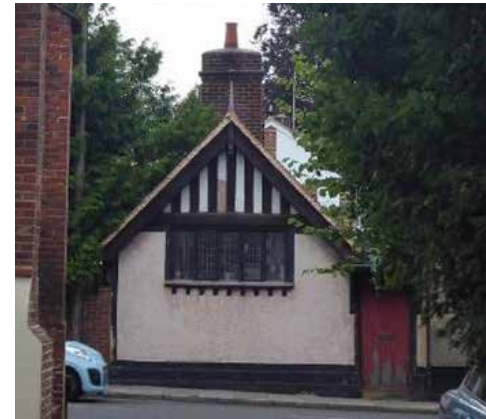
Figure 51 37A Bradford Street
