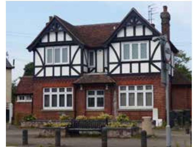
Figure 56 The former Six Bells Public House
