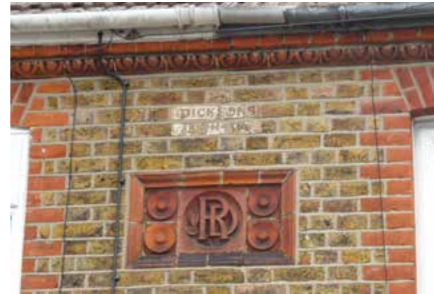
Figure 92 Example of decorative brickwork
