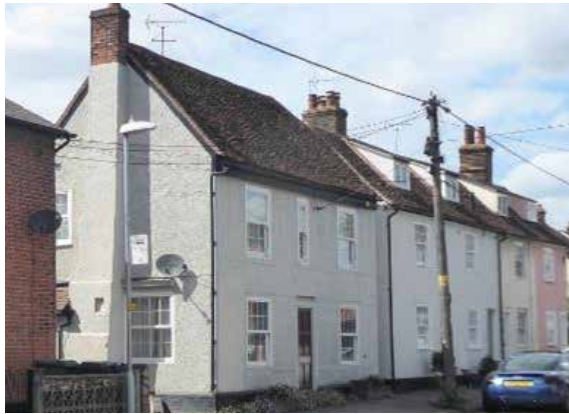
Figure 57 The former Spread Eagle Public House
