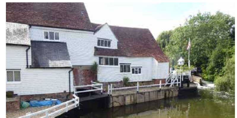
Figure 74 The view west, looking over the bridge toward the mill
