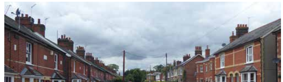
Figure 91 Roofs on Woodfield Road
