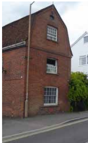
Figure 81 Red brick, South Street
