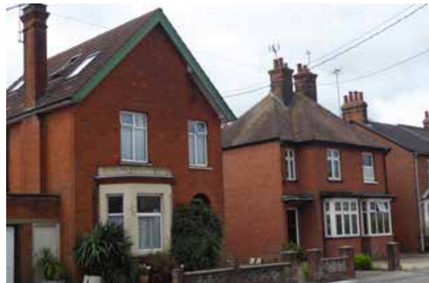
Figure 109 Examples of red brick and gardens removed to facilitate off road parking, Rayne Road
