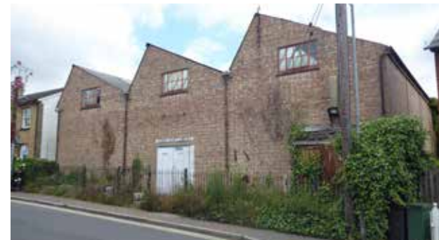
Figure 79 Saw-tooth roof, otley Road
