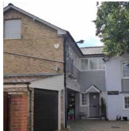
Figure 29 Former nineteenth century printing works behind 85 Bradford Street
