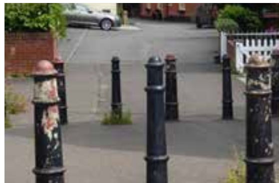
Figure 83 Bollards in Woolpack Lane
