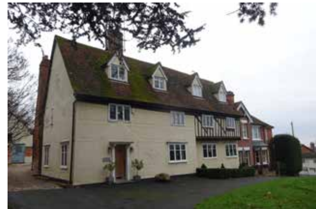
Figure 14 Example of pargetting, exposed timber framing and brick work at Ivanhoe House
