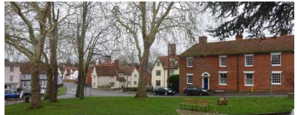
Figure 16 Various window types and materials are present on The Green, yet the use of traditional materials and construction creates a unified appearance
