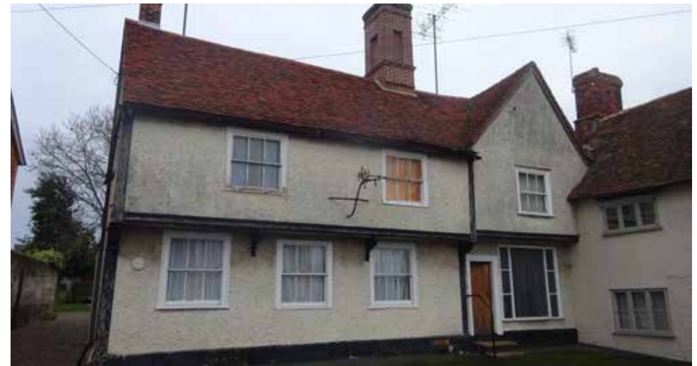
Figure 23 Castle House, High Street
