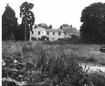
Figure 40 North elevation of the Hall 1984 (ECC)
