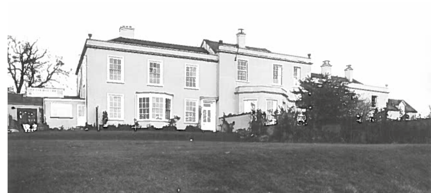
Figure 47 South elevation of Manor House [nd] (ECC)
