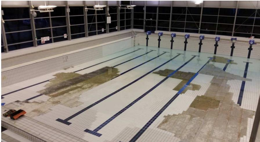
On Monday 27<sup>th</sup> February 2017 preparation works started on Braintree swimming pool to reline the pool tank. Two submersible pumps were dropped in to the pool to drain the 630 cubic meters of water. The pool took seven days to empty and works have now started on removing the tiles from the pool tank. Once the concrete has dried sufficiently the epoxy resin coating will be applied. The pool is due to re-open towards the end of April 2017.
